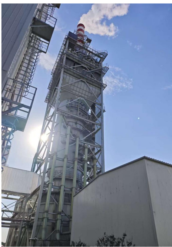
SNCR+SCR 脱硝+石灰-石膏法脱硫+湿电除尘器+78m 排气筒 DA003
