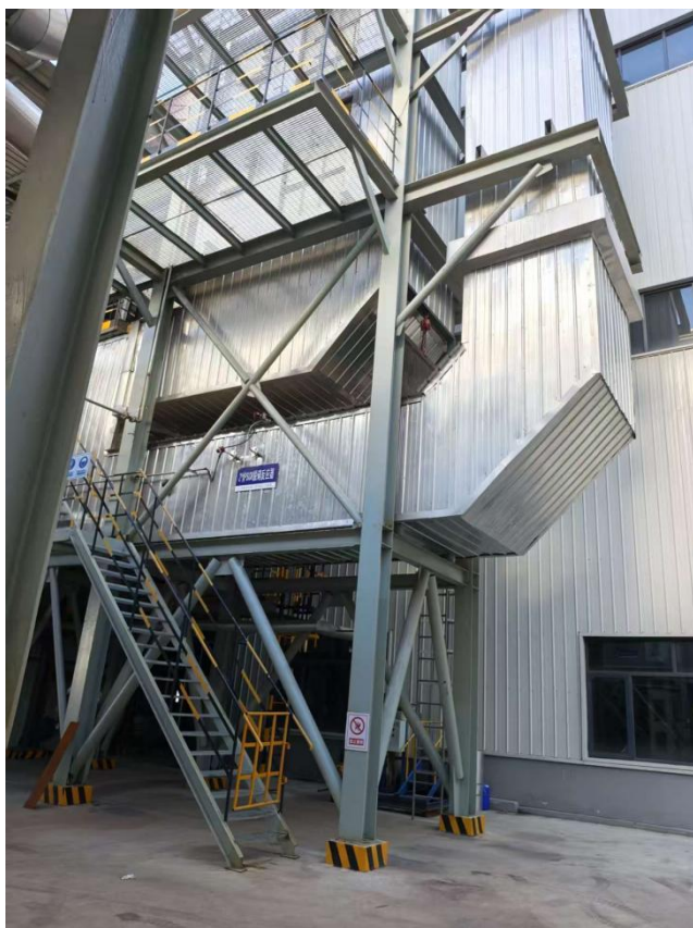
SNCR+SCR 脱硝+石灰-石膏法脱硫+湿电除尘器+78m 排气筒 DA003
